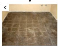
a. If the underlayment substrate plywood is less than 3/4" thick or is a wood product other than plywood, add a second cross layer for strength and stability not less than 5/16" thick. To prevent squeaking, use ring shank nails, coated nails or coated staples every 6" to secure the second layer. Glue (construction adhesive) and screw down plywood, when installing any added layers of plywood to the subfloor.
